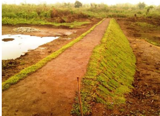
5 check dams were built – some with mud and some stone and concrete. Total cost was around 7 lakh rupees and we hope it will benefit 150 farmers directly apart from recharging the wells which now remain dry 6
