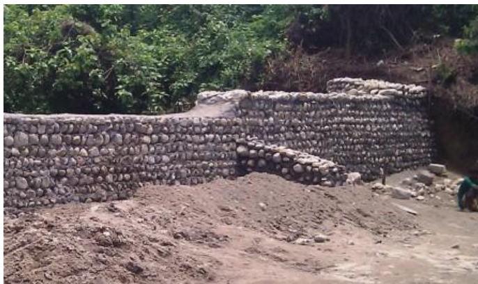
5 check dams were built – some with mud and some stone and concrete. Total cost was around 7 lakh rupees and we hope it will benefit 150 farmers directly apart from recharging the wells which now remain dry 6
